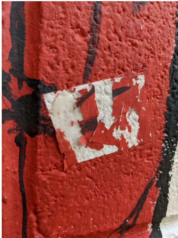
Mural Damage, Close-Up (peeling paint located 2 ft. 2 in. above floor)
